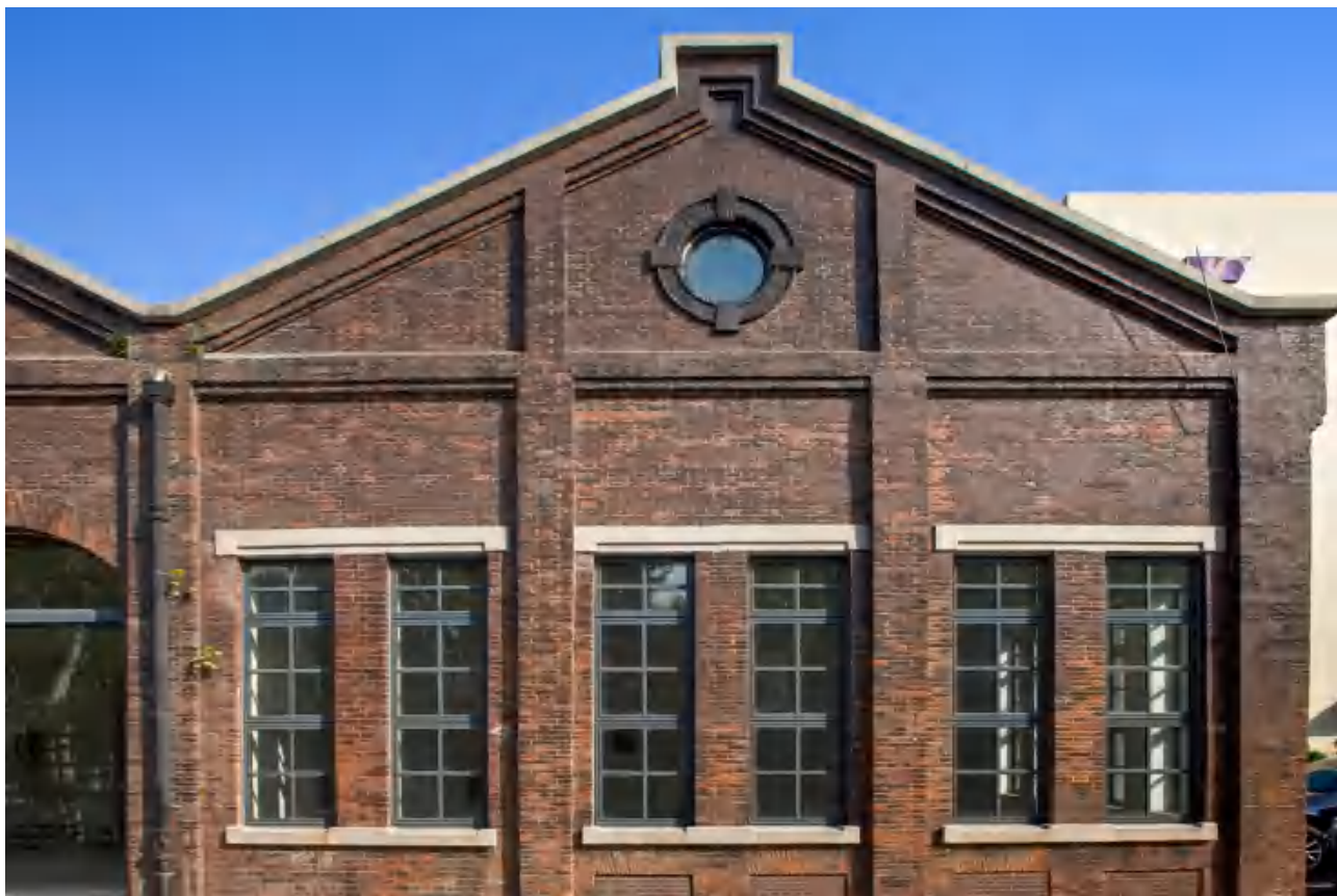
修旧如旧的山墙 Left: Repairing the old gables
