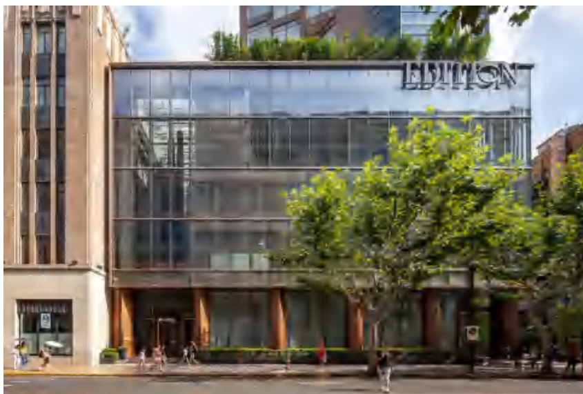
新建裙房立面实景 On-site View of Completed New Podium (After Renovation)
